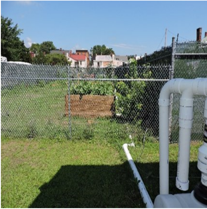
Photo C. Pipe connecting the rainwater collection and first flush components to the raised beds. The rainwater travels through the pipes due to the gravity of the slight downward slope.
